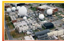
Scramjet Test Complex
