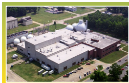
4-Ft Supersonic Wind Tunnel
