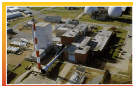
8-Ft High Temperature Tunnel
